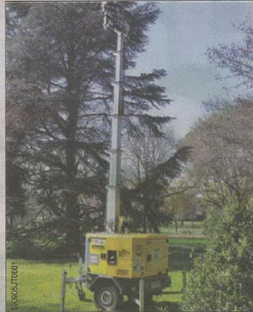
DAMAGED: Unknown offenders have vandalised flying fox dispersal equipment at the Colac Botanic Gardens less than 24 hours after the program began.
